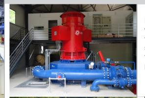
Pelton turbines are suitable for high heads and small flows and with a wide range of configurations appropriate for a different turnkey project supplies. Siapro uses standardised manufacturing process to secure high quality of the end product. We offer consulting, engineering services, production and implementation.
